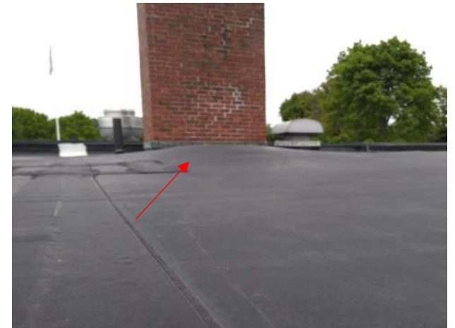
12. There are areas where the roof has bubbled and the membrane is no longer adhered.
