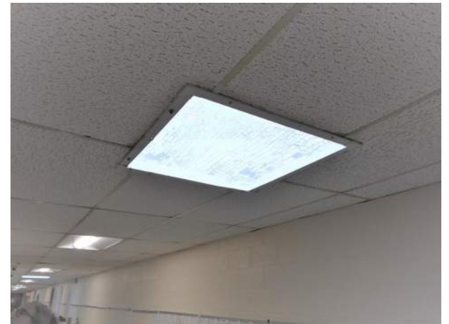
18. The skylights in the corridors are damaged.
