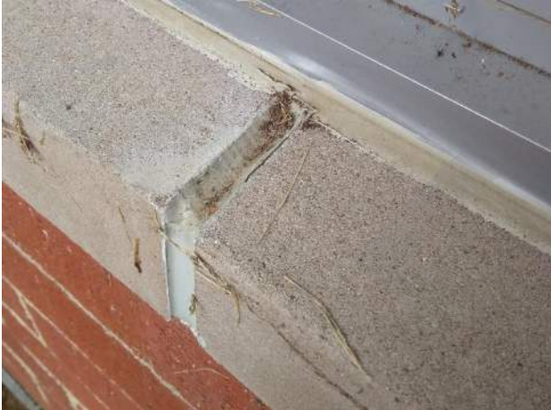
4. Some sealant shows early signs of deterioration.
