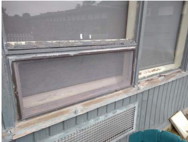
2. Original windows and trim have deteriorated.
