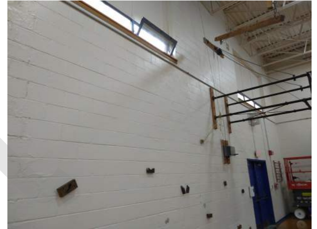
15. The brick/CMU wall of Gym shows signs of extensive water damage and is not insulated.
