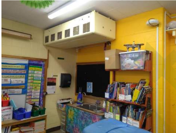
20. Classrooms have outdated and inefficient unit ventilators.
