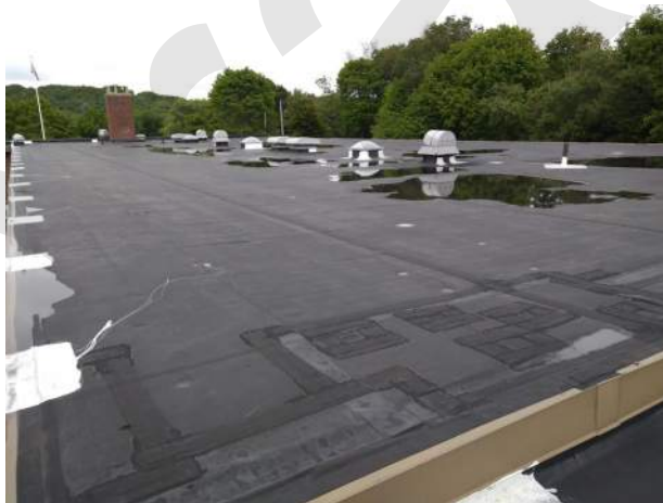
11. Rubber membrane roof has many areas of standing water and is extensively patched.
