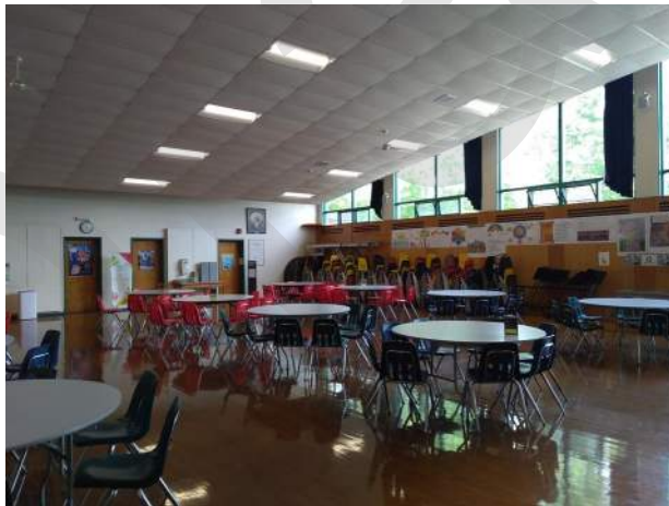
17. Existing 2x4 ceiling tiles have sagged and are cupped.
