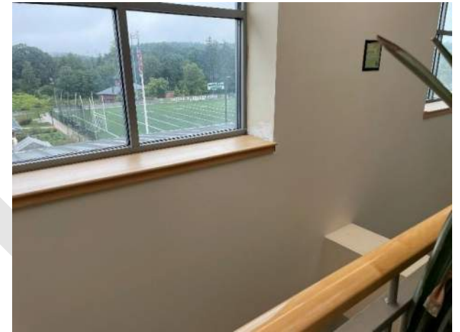
9. Several windows show signs of water damage.
