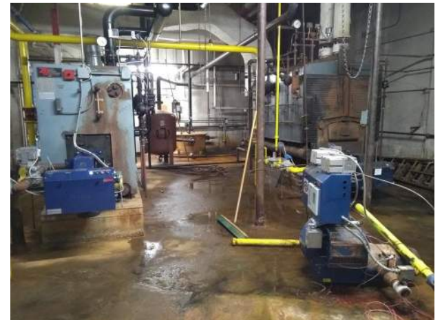
30. Boiler room shows signs of chronic flooding, equipment is obsolete and inefficient.
