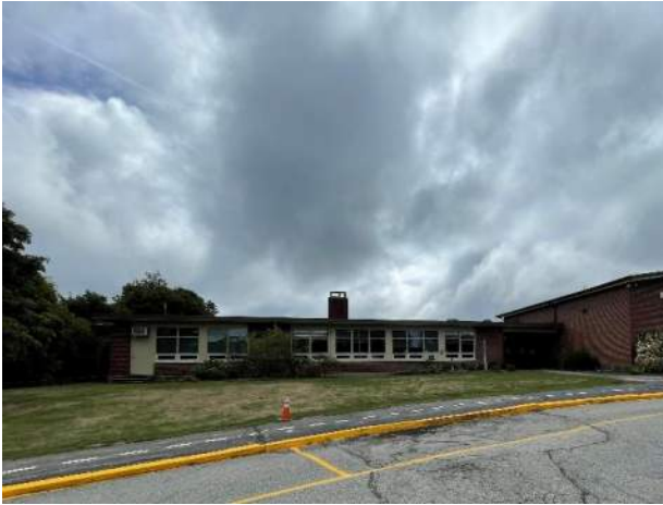
1. Bituminous driveway shows signs of cracking and freeze/thaw damage.
