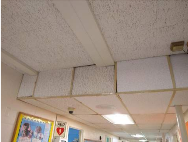
19. Existing 2x4 ceilings are discolored and tiles are mis-matched.
