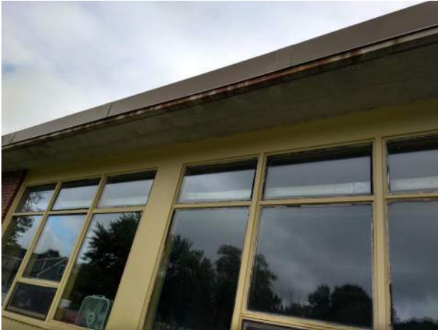
7. Original roof soffits have corroded.
