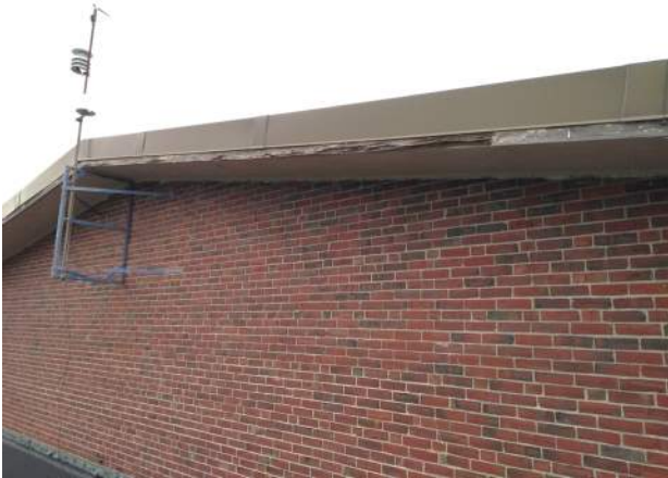
13. The fascia is rotted at the Cafetorium.
