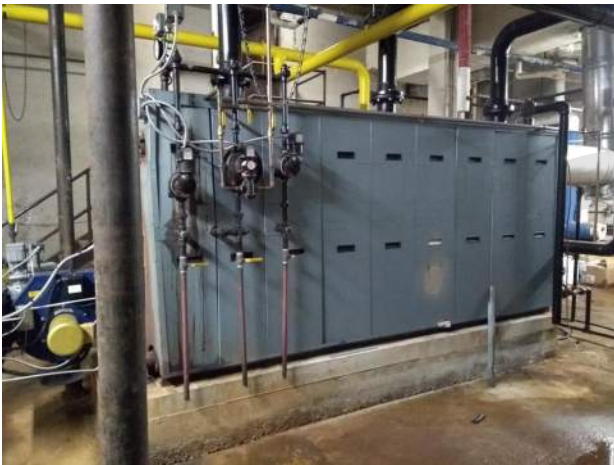
28. This boiler was installed in 2008 and still functions.
