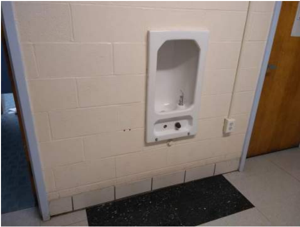
25. All drinking fountains are original and are not AAB compliant.
