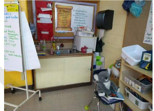
21. Classrooms have outdated sinks that do not meet AAB accessibility requirements.
