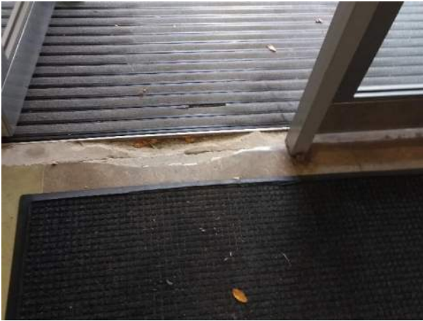
7. Threshold at entry is damaged. Walk off matt is worn.
