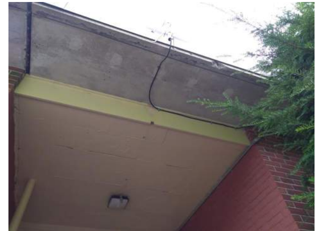
6. The concrete fascias and soffits have spalled.
