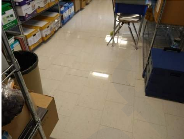
14. Vinyl floor tiles in Modular addition show signs which may indicate issues with subfloor.
