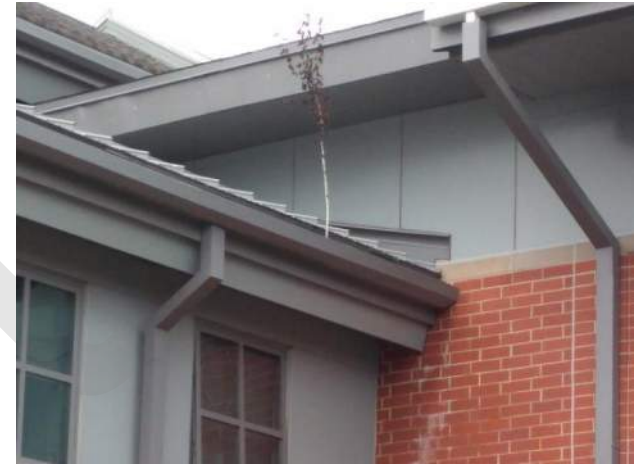
3. Some gutters are clogged with vegetation.
