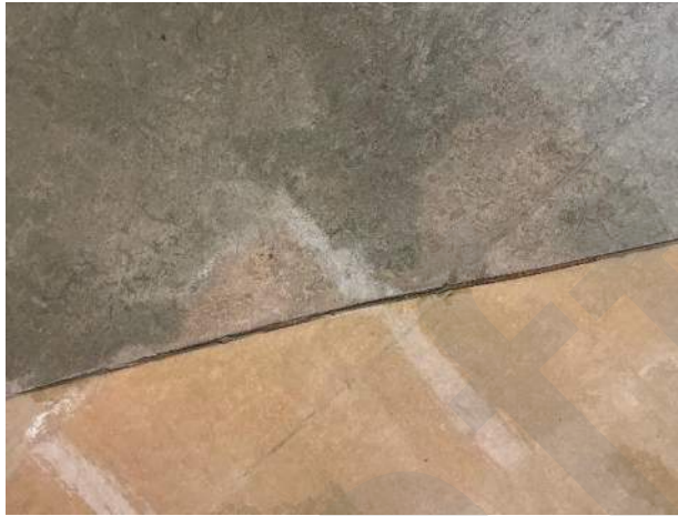
8. Some floor joints at natural linoleum are damaged.
