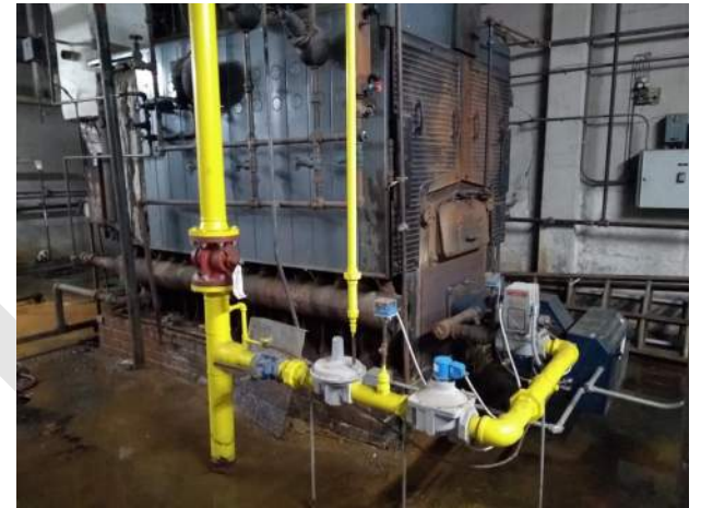
27. This 1975 era boiler is no longer being used.
