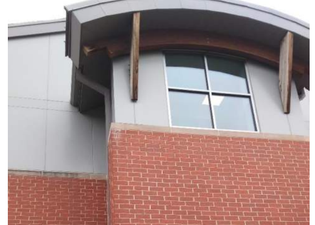
6. Discoloration is evident at wood accents, brick and precast.
