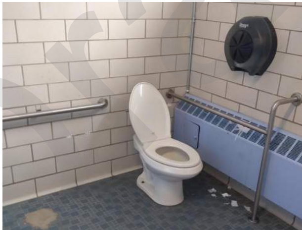
23. Grab bars/accessories are non-compliant and original tile floor is patched.
