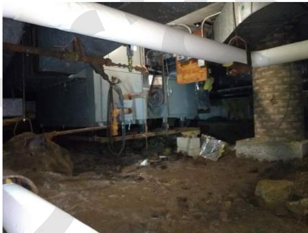
29. This Air Handling Unit in the crawl space is obsolete.
