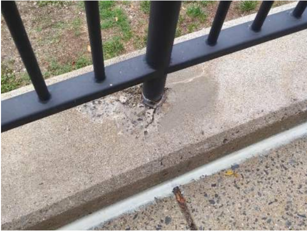
1. Concrete has spalled at some rail posts.
