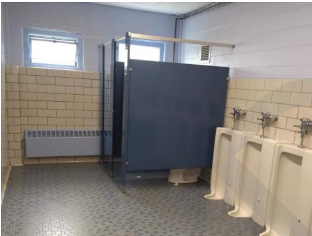
22. Multi-user toilet rooms have original, outdated fixtures and several have no AAB updates.
