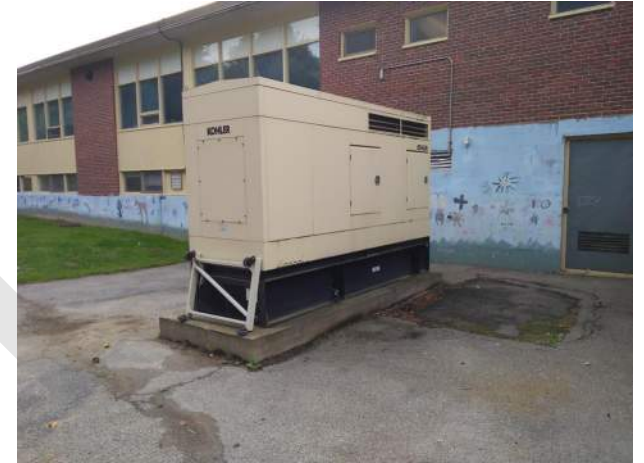
9. Confirm that generator has been maintained per manufacturer's recommendations.
