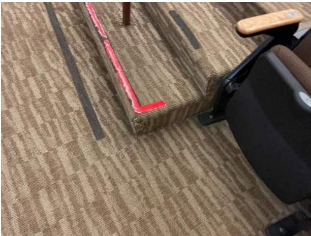
10. Original carpet at Auditorium is showing signs of wear.
