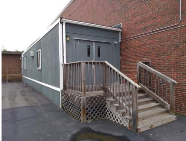
8. Modular addition has deteriorated and leaks at connection to main building.
