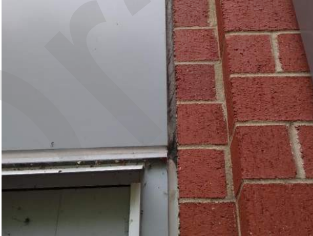
5. Sealant at metal panel is showing signs of deterioration.
