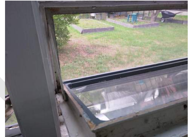
3. Operable steel hopper window has no weather strip.
