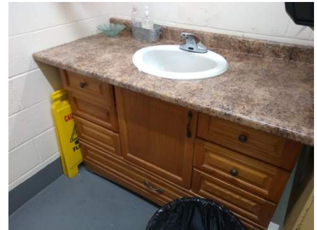
24. Single-user toilet rooms do not meet AAB requirements.
