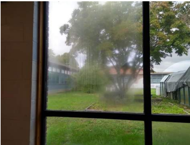
4. Thermal pane window has seal failure.
