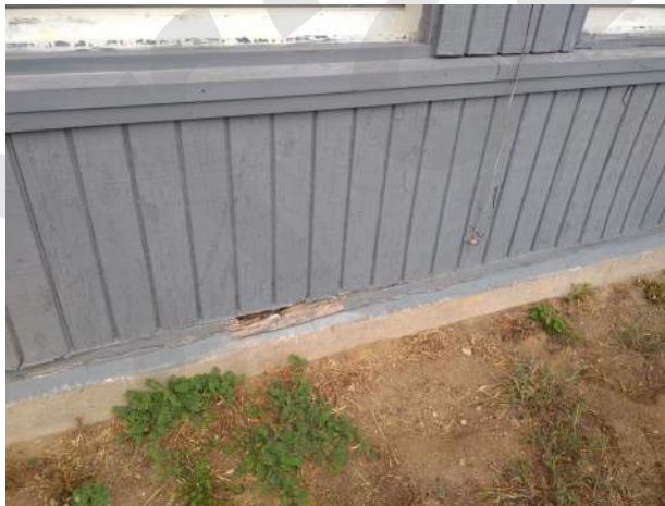
5. The wood siding is rotted and damaged.
