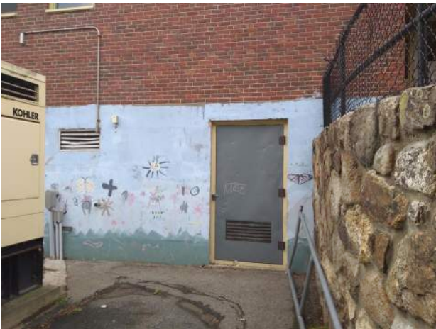
10. Bituminous pavement is damaged, original hollow metal doors require repair/replacement.
