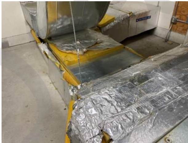
11. Some duct work has damaged or missing insulation.
