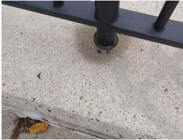
2. Rail posts do not have sealants and some sealants are failing.
