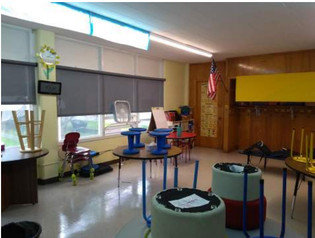
16. Classrooms have outdated spline ceiling and insufficient ventilation.
