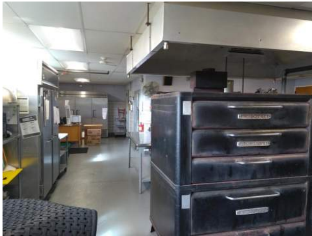
26. Kitchen equipment is very old and inefficient.
